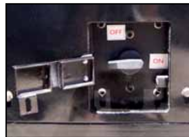
Lockable dual pole battery isolation selector for safer maintenance note: can only be locked in off position.
